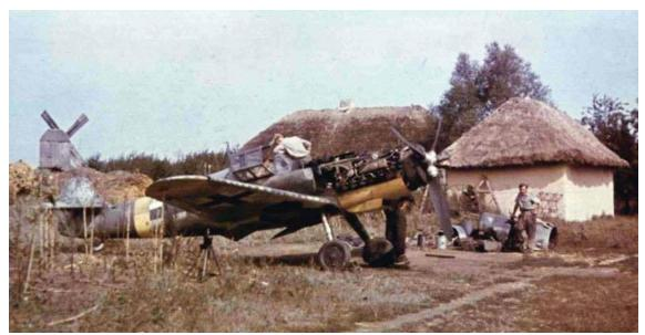
In this rare color photograph, an aircraft believed to be an Me-109 of JG 52 undergoes repairs somewhere in Russia. German maintenance crews struggled mightily to keep their planes in the air due to shortages in spare parts and fuel.
