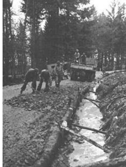
Engineers repairing a muddy road in the Hürtgen Forest
